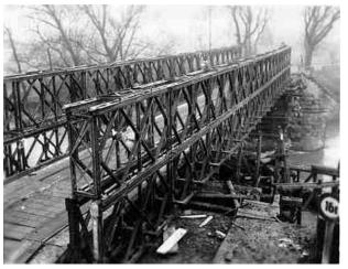
*An example of a Bailey bridge constructed by Combat Engineers.*
