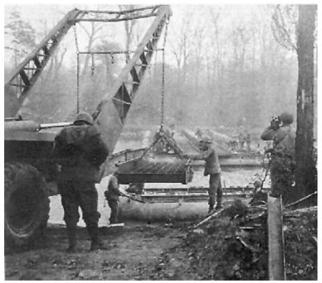
Combat engineer troops position the heavy steel treadways, measuring approximately 12 feet in length, using a crane truck. This operation is performed on the near side, or "friendly side", of the river.
