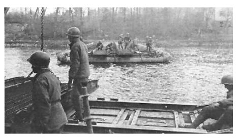
Two steel treadways are pinned across each ponton. The treadways are spaced to fit the tread widths of tanks, tank destroyers, trucks and other vehicles. After the steel treadways have been attached to the ponton, the section is then tied to the bridle line, pushed across the river, and pinned to the previously constructed bridge sections. For added stability, bridge anchors, much like boat anchors, are dropped upstream of each ponton.
