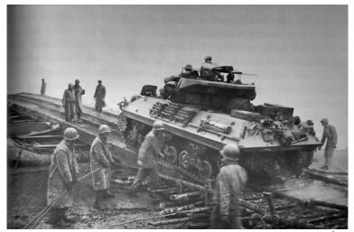
A tank destroyer is loaded onto an infantry support raft in the 358<sup>th</sup> Infantry sector by Combat Engineers of the 206<sup>th</sup> Engineer Combat Battalion. Notice the corduroy road constructed to the edge of the Saar River to prevent vehicles from sticking in the mud.
