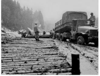
Combat Engineers construct a section of corduroy road. Corduroy road is constructed from poles cut from the woods and laid in mats to permit vehicles to travel along muddy roads.
