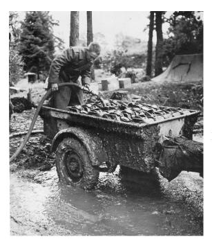
Five-gallon water cans loaded on a quarter-ton trailer being filled at an Engineer water point. The Engineers were responsible for the purification of drinking water and set up water points from which all units located in the area drew their daily supply.
