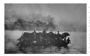
Three (3) types of ferries were used. Infantry support rafts carried weapons carriers, jeeps and anti-tank guns. Class 40 ponton<sup>2</sup> ferries transported medium tanks and tank destroyers across. Then, storm boats and assault boats, powered by out board motors, and powerboats carried rations and ammunition to the far shore and returned with wounded.
