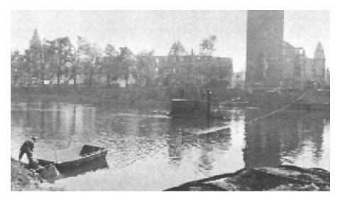
A bridle line, normally a one-inch cable, is stretched across and anchored on both sides of the river. The bridle line, located upstream of the intended position of the treadway bridge, is used to hold the bridge in position. Other preparations include the grading of approaches to the bridge and may also involve the construction of corduroy road or other site preparation, depending on soil and weather conditions.
