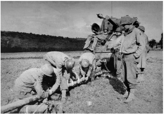
Combat Engineers assemble a "Snake" demolition to be launched by an M-4 tank.
