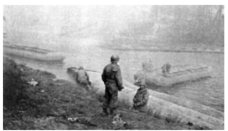
The pontons are inflated and readied for bridge construction, normally in a location sheltered from enemy fire and, if possible, out of the currents of the river. They are then either floated or hauled by truck to the bridge site, depending on where these preparations are made.
